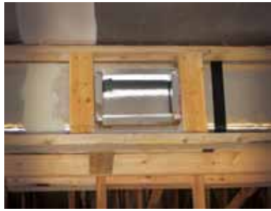
Small, one-level homes can be served by a single main duct chase running through a dropped ceiling in a central hallway. Short sheet-metal ducts can be fashioned on site to direct air into each room off the hall.
