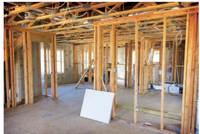
These insulated ducts are on joists with centrally located supply registers showing, but these are open-web floor joists—not attic roof trusses. PHOTO: COURTESY BUILDING AMERICA
