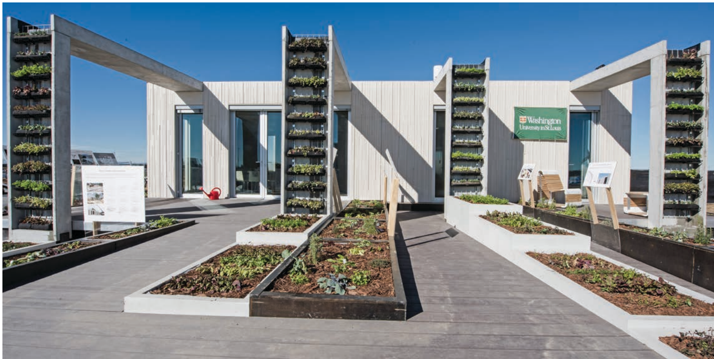
CRETE House, a joint entry from the University of Washington and the Precast/Distressed Concrete Institute, measures 995 square feet. It highlights the disaster resiliency offered by building with factory-made exterior wall panels that are assembled onsite.
