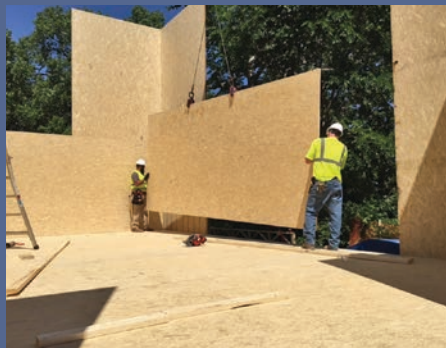
At a Habitat for Humanity project in Minneapolis, a Monopath tall wall is installed.
