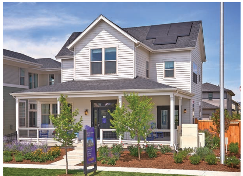
Thrive's Vita Collection models at Stapleton include finished basements and big pantries. They're the first homes in which the builder installed energy recovery ventilators (ERVs). The homes range from 1,798 to 2,566 square feet.
