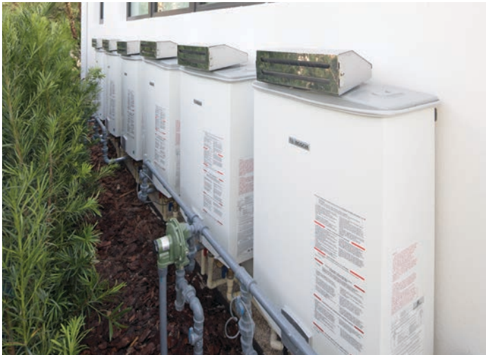
From the top: The 60-panel solar array can put out 17 kW; two Tesla Powerwall batteries store solar energy and lessen the nighttime load on the house; six Bosch tankless water heaters ensure there's plenty of hot water available throughout the house, whose total area is 12,509 square feet.
