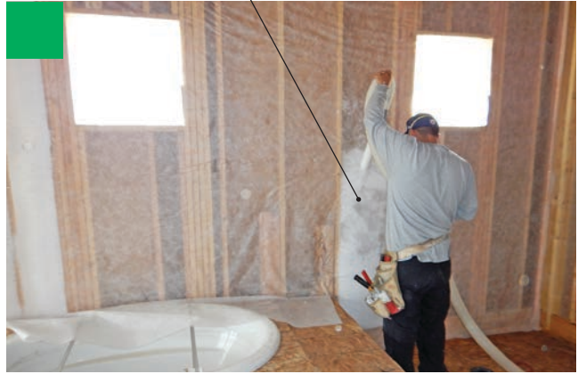
Inadequate insulation in a 2x6 wall cavity can be rectified with blown insulation.
