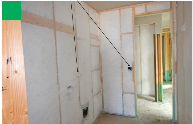
Blown insulation ensures proper fill around pipes, wires, electrical boxes, and any other obstructions.
