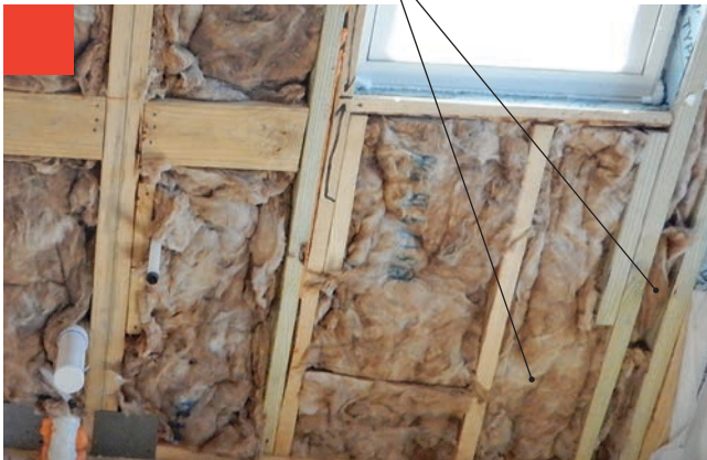
Odd-size cavities can be insulated with consistency using blown insulation.
