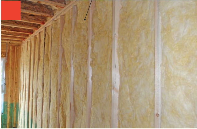
Inadequate insulation in a 2x6 wall cavity can be rectified with blown insulation.
